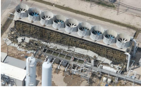
Tower Structural Failure
